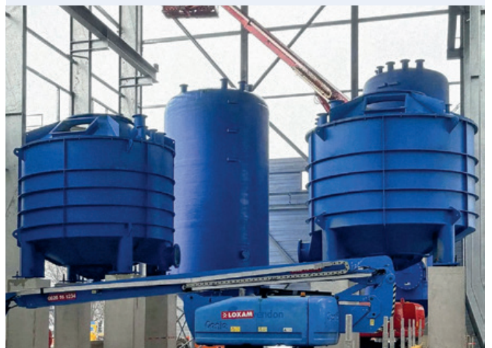
BTA pre-treatment in Gennevilliers during installation
